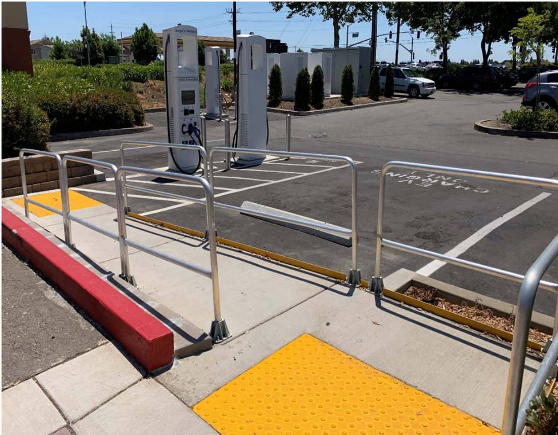
Electrical vehicle charging station on an accessible route - Photo taken by Juvoni Sterling
